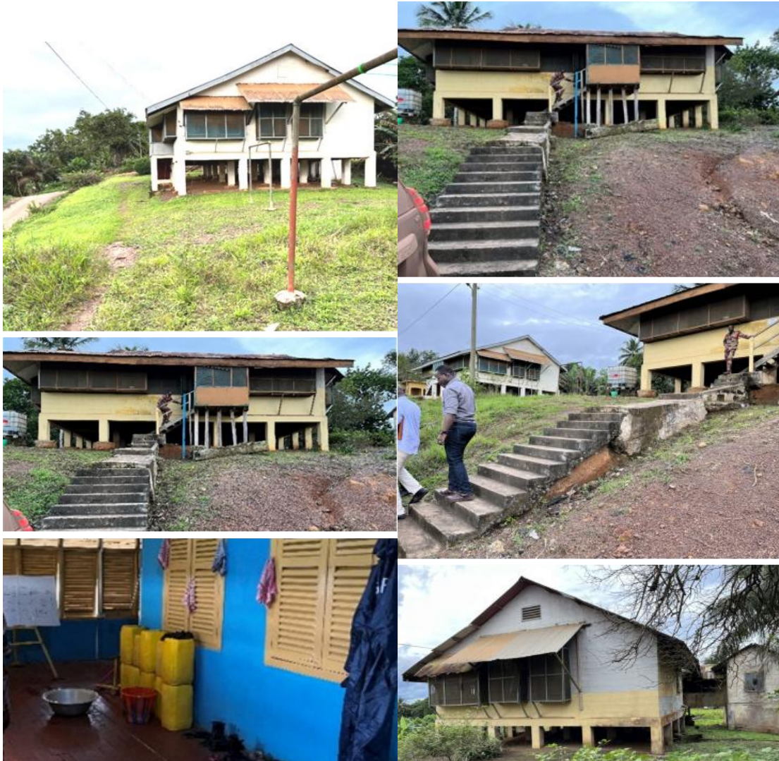
Figure 1 Photos of back and front views of the Prestea building Location of Prestea Office Facility in the Western Region
