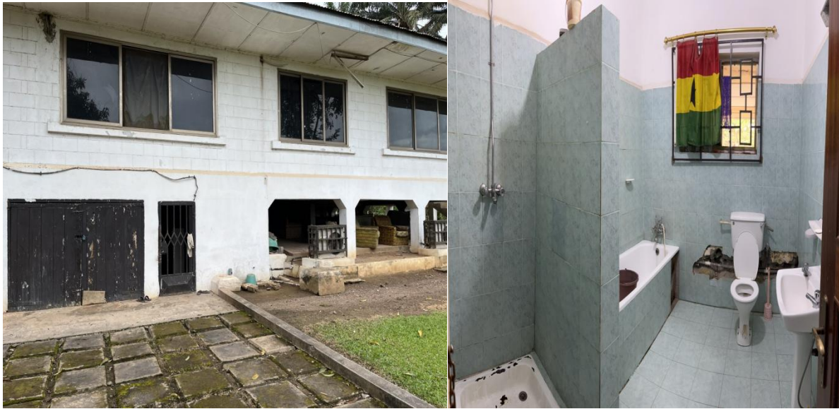
Figure 1 Photos of back and front views of the Tarkwa building
